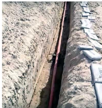
Figure 1: Displayed the Direct Laying Procedure.
