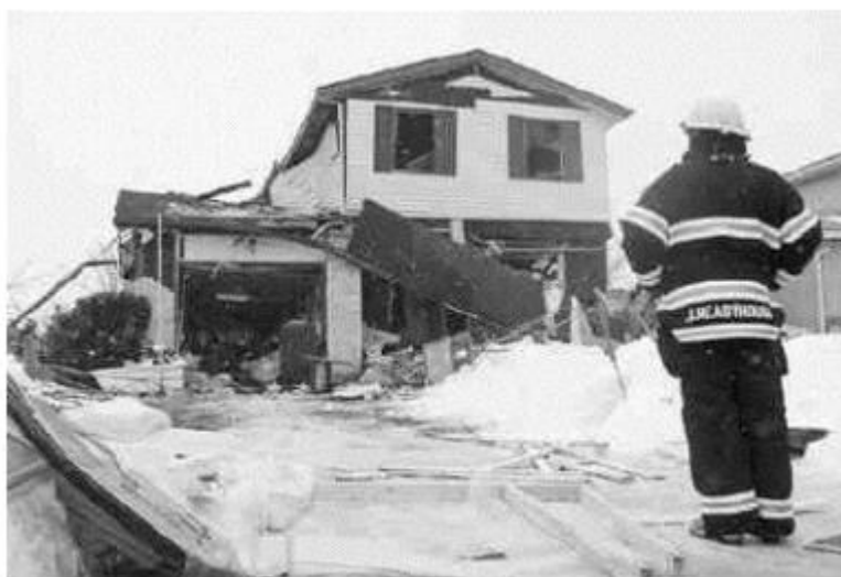
Figure 1: Damage that occurred due to LPG explosion.
